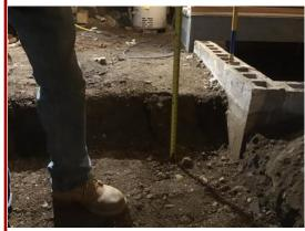
In anticipation of the third balcony being built, secure footers were added in the basement to hold the weight of the library's nonfiction collection, as well as some of the stacks. Neither
